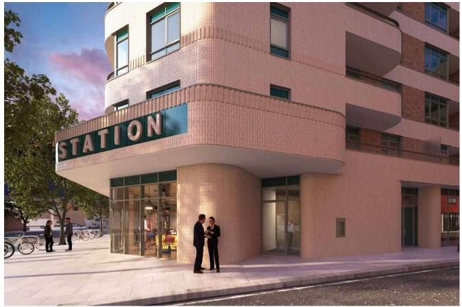
CGI image showing the vertical soldier course brickwork and projecting 'dentil' brick course at window cill and canopy cornice level
